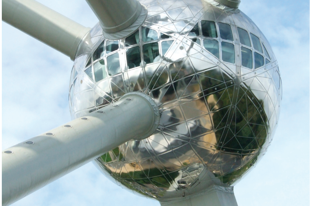
Photo 2: Atomium Brussels. The renovated spheres are now clad with sandwich panels made of 1.2 mm outer skin of X2CrNiMo17-12-2/t.4404 stainless steel grade – Brussels (B)
