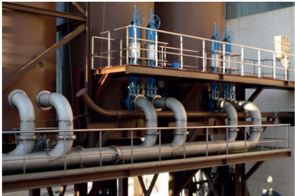
Mud dehydration entry to storage silo Photo: Cedinox, Madrid (E)
