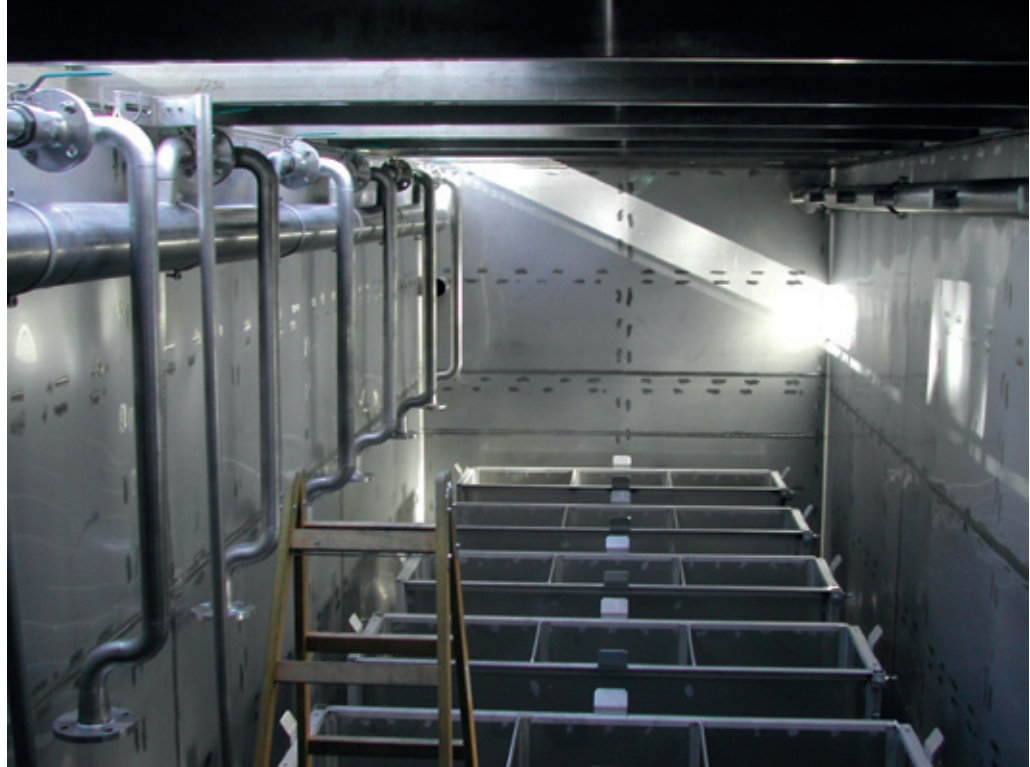
Inside the container with membrane housing stainless steel boxes Photo: Centro Inox, Milan (I)
