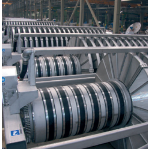
Micro-strainers for the removal of finely suspended solids from the secondary clarifier's effluent
