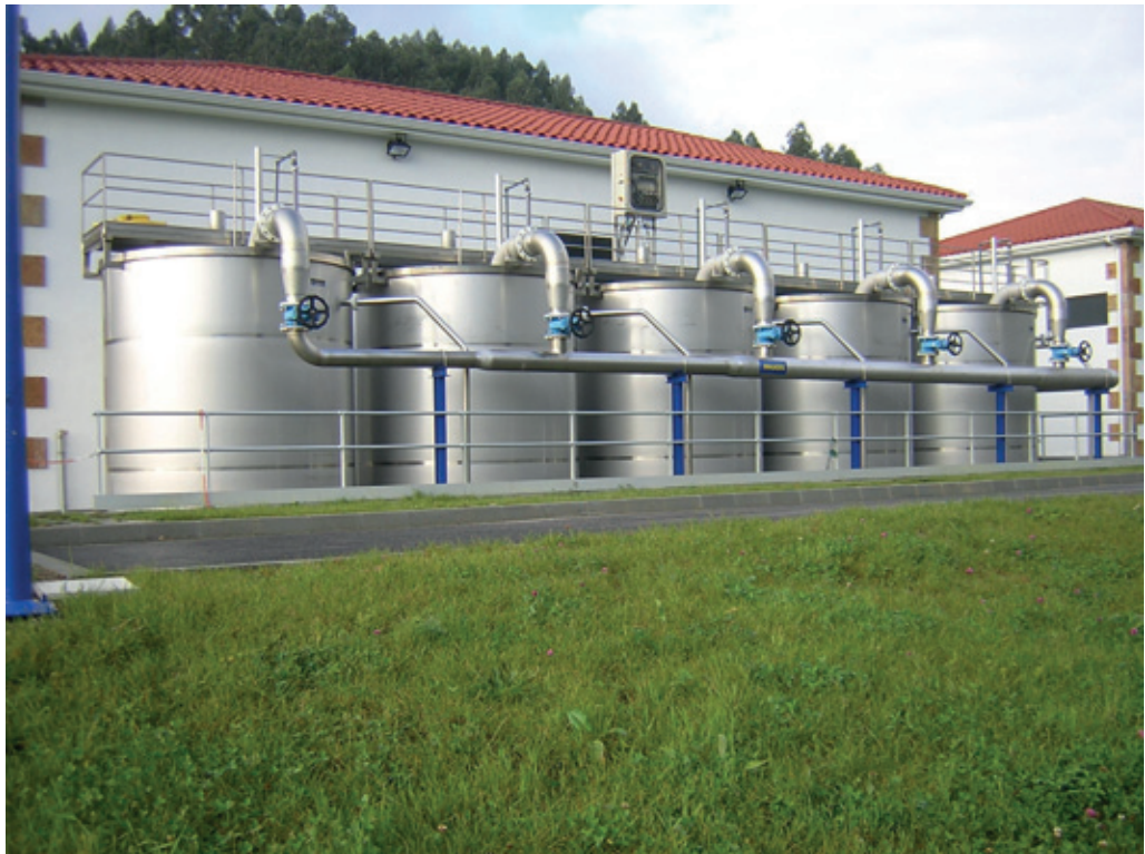
Stainless steel containers and piping in a waste water treatment plant Photo: Hans Huber, Berching (D)
