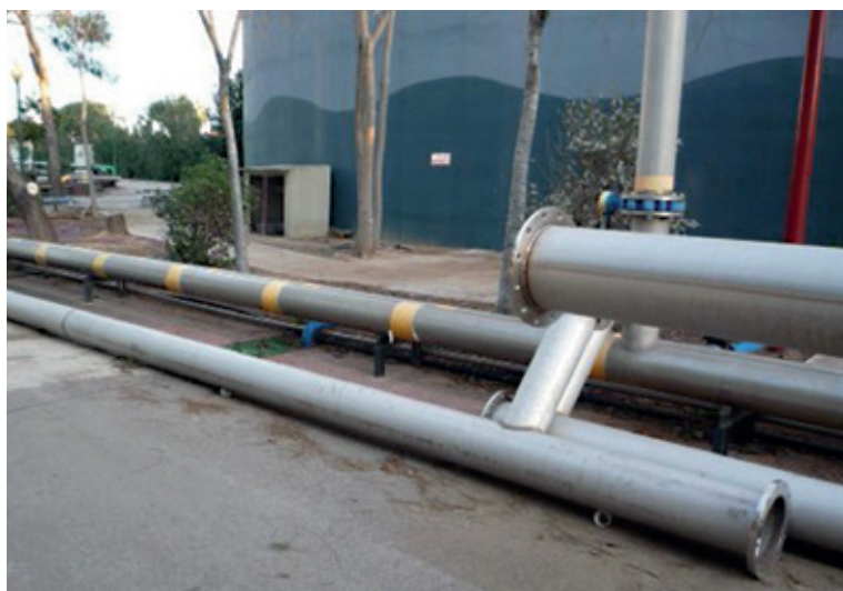
Pipe systems before assembly in a sewage plant Photo: Cedinox, Madrid (E)
