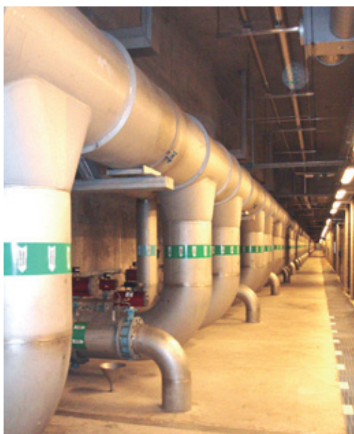
Piping system below the sandfilter basins in sewage treatment plant in Stockholm (S) Photo: Outokumpu, Avesta (S)
