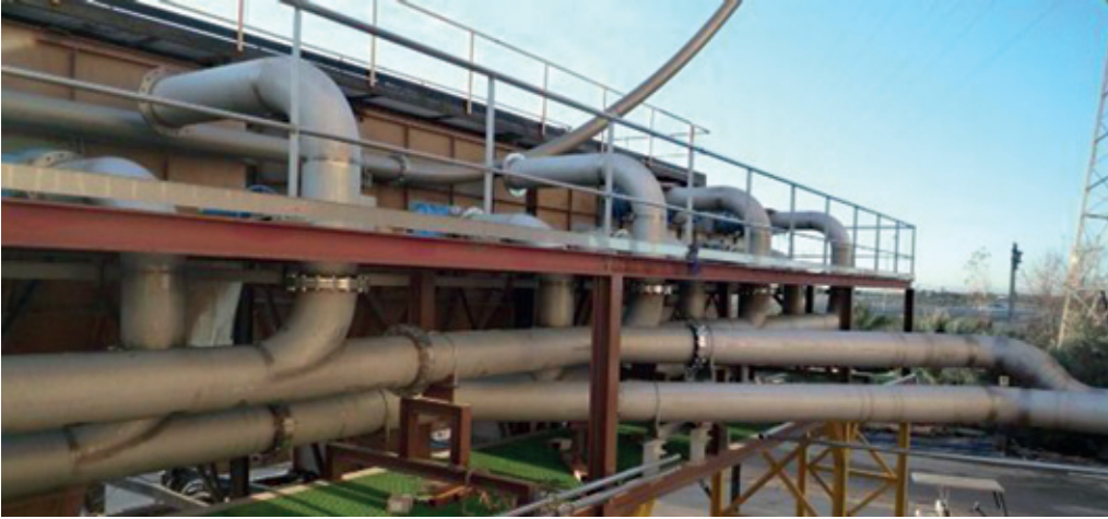
Sectional view of the waste water treatment plant with stainless steel pipes and railings Photo: Cedinox, Madrid (E)
