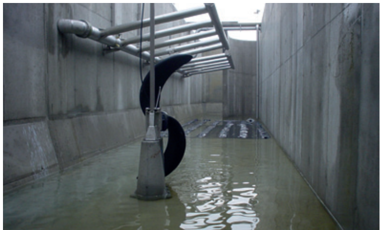
Detail from waste water treatment plant Photo: Regeneracija, Lesce (SI)
