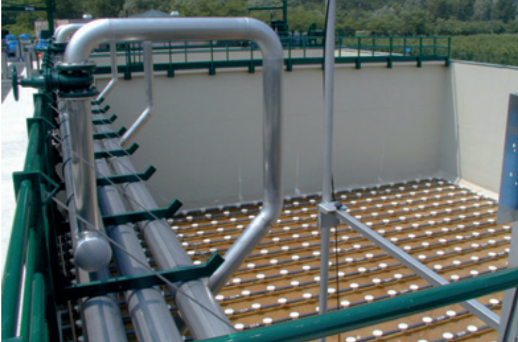
Bare and painted stainless steel surface is used in Lavis (I)
