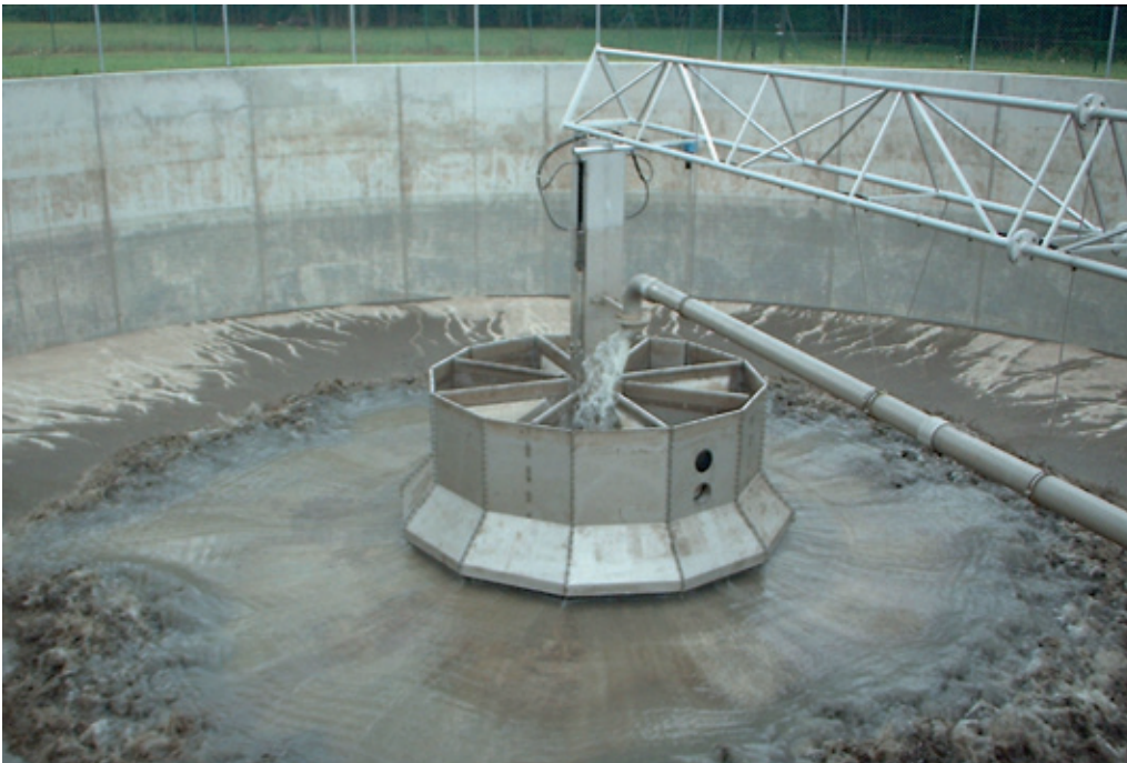
Round tank flushing system – wave flush for circular and small rectangular tanks Photo: Steinhardt Wassertechnik, Taunusstein (D)
