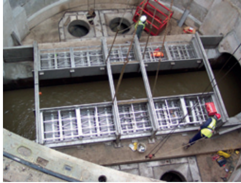
Fine bar screen for water pollution control in case of emergency discharges and its installation in a sewer overflow Photos: Steinhardt Wassertechnik, Taunusstein (D)
