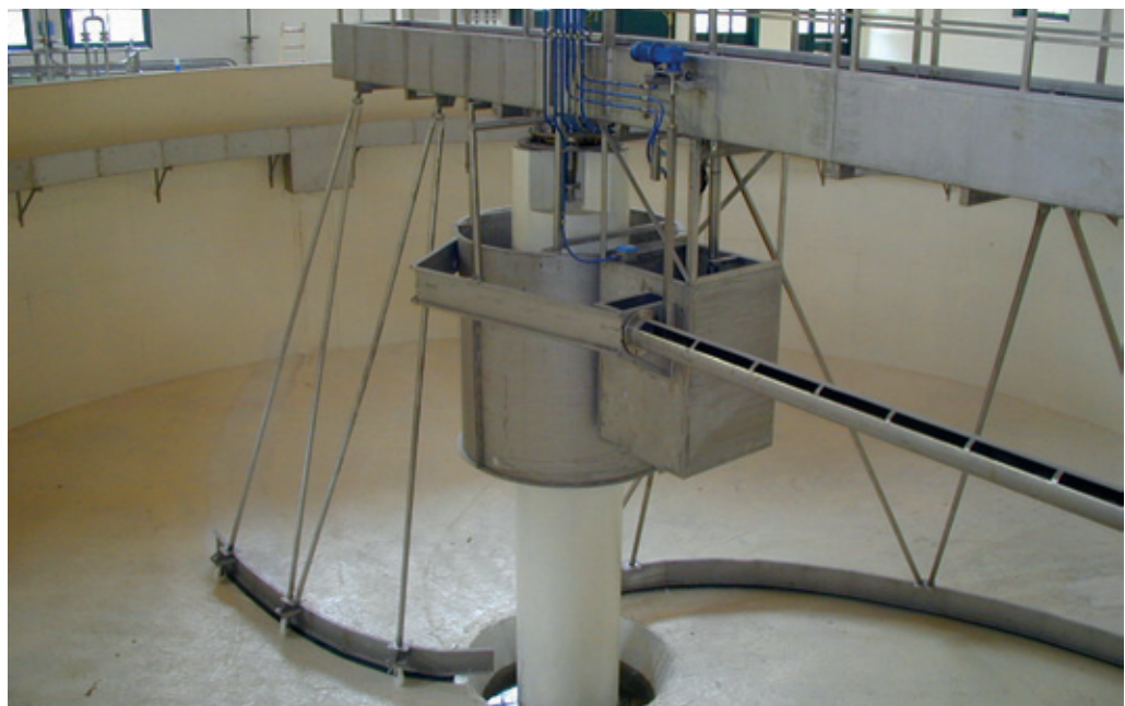
Completely roofed purification plant in Val- larsa (I) Photo: Centro Inox, Milan (I)
