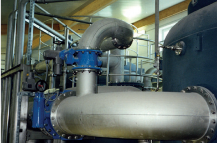
The selection of material for pipes helps to reduce costs in the construction Photo: H. Butting, Knesebeck (D)
