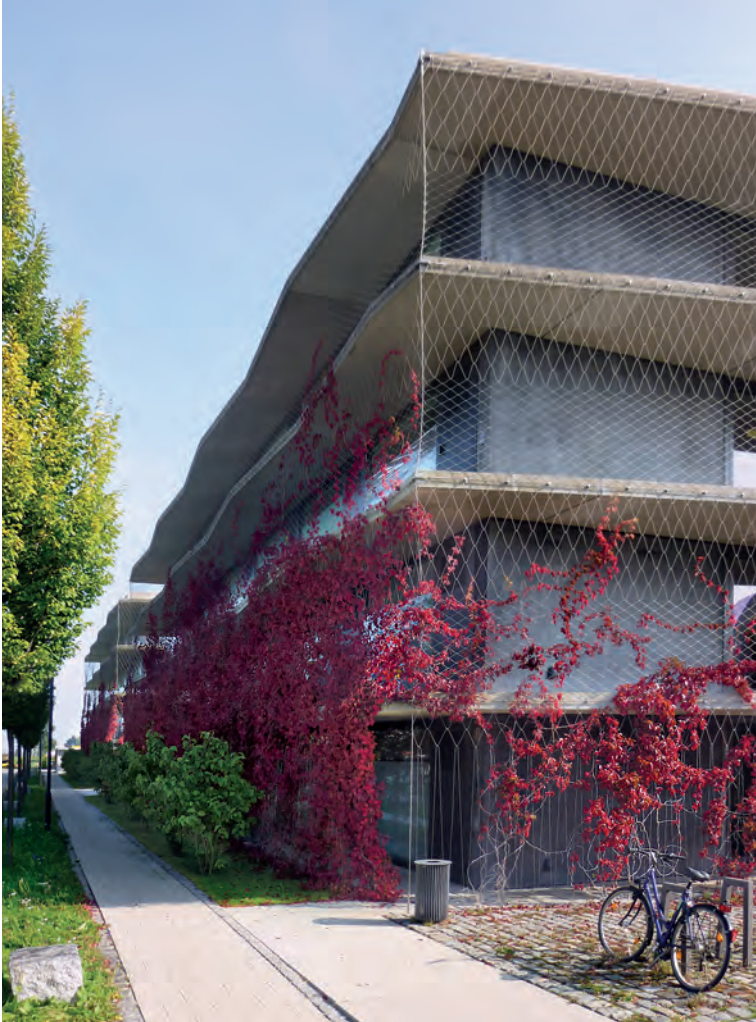
The cable net and the vegetation growing up it wrap around the outside of the cantilevered floor slabs.
