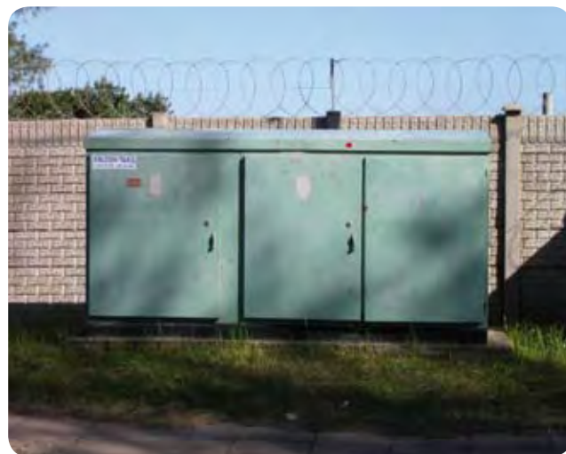
Electrification box, in painted grade 410, S. Africa.
