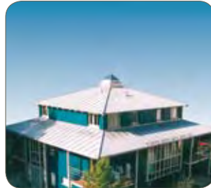
Grade 1.4510/430Ti (standing-seam technique), Ugine & Alz, Germany.
