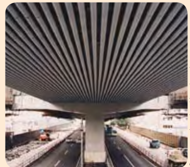
Overpass noise-absorbing plate, Japan.
