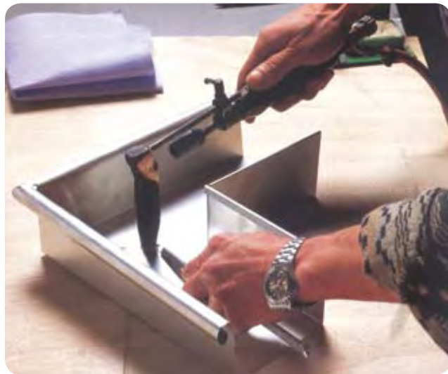
Soldering a gutter, tin-coated grade 430Ti.
