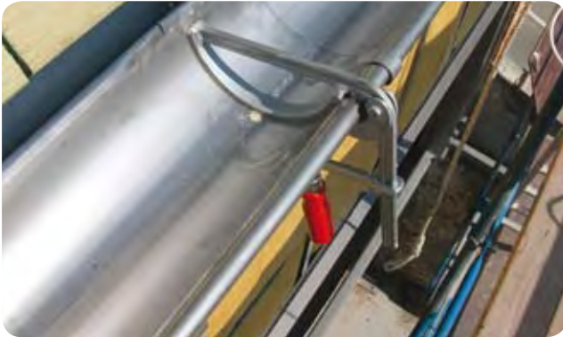
Bonding of guttering, tin-coated 430Ti.
