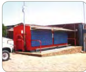
Grade 1.4003/410, painted, SASSDA, South Africa. "Utility" ferritics are often painted, when aesthetic considerations are important.
