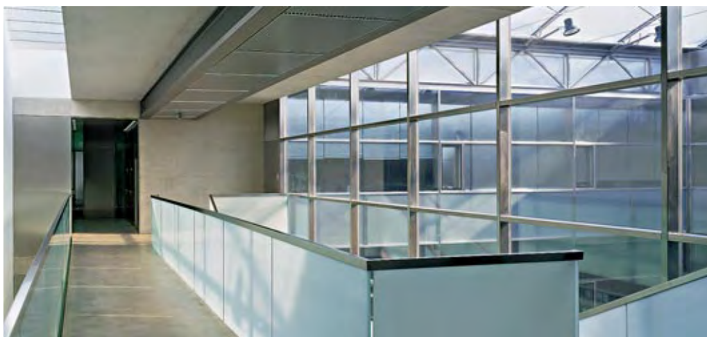
The inner courtyard has a slim post-and-rail façade of stainless steel profiles and insulating glass. The glass balustrades are matt finished.
