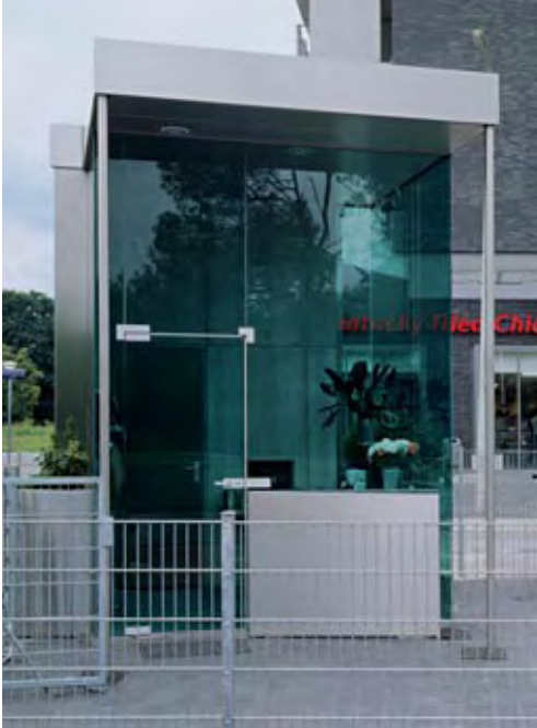
The large, low-maintenance surfaces of tinted green glass and stainless steel emphasise the exciting shape of the bikehouse, created by simply offsetting two interpenetrating square volumes in relation to each other.
