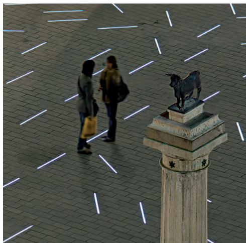
A casing of 2 mm stainless steel sheet (EN 1.4304) and a covering of laminated glass protect the lighting strips fitted flush into the basalt pavers on the square.
