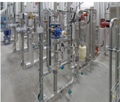
In hospitals, plumbing systems must withstand common disinfection procedures. Photos: Nussbaum, Olten (CH)
