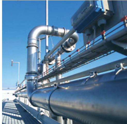
Stainless steel press-fit fitting systems are also suitable for a wide range of chemical products. Photo: Raccorderie Metalliche, Campitello di Marcaria, MN (I)
