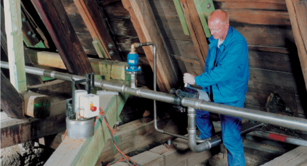
As a fully mechanical type of joints, press-fit connections are produced at ambient temperature and any fire risk is avoided. Photo: Geberit, Jona (CH)
