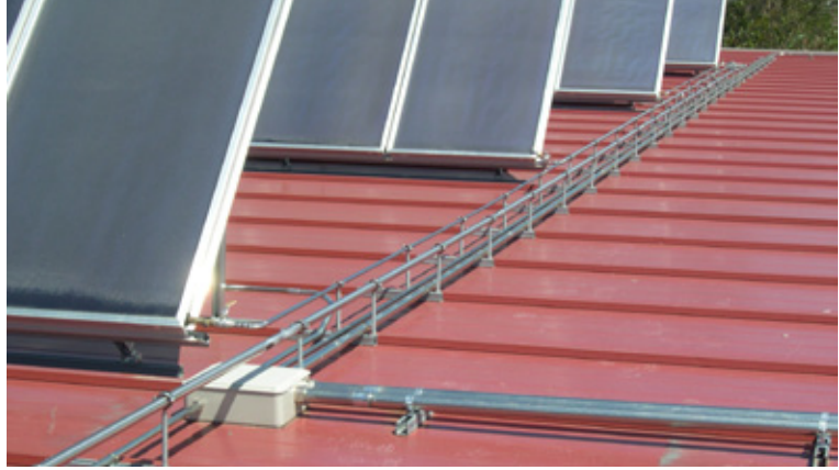
Insulation materials and clamp inserts, which come into direct contact with stainless steel, must not release any chlorides. Photos: Filtube, Barcelona (E)
