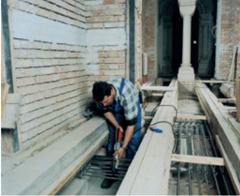
In the retrofitting of heating installations in listed buildings, the advantages of a cold process, which does not involve any fire hazards, are particularly appreciated. Photo: Geberit, Jona (CH)
