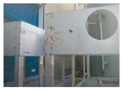
Contamination of stainless steel by iron: the example displayed is a typical case of iron contamination caused by the mixed use of iron (or steel) and stainless in the same shop without proper materials segregation. In the process of decontamination, it is important that the traces of iron are really removed and not just spread.
