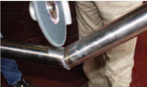
Treatment of the inside angle with an internal angle finishing tool
