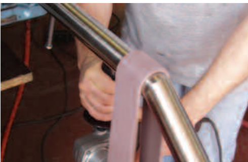
Finishing operation with an easy-to-use powered hand-held tool. The sharp angle of the joint is still visible with the weld fully blended in.
