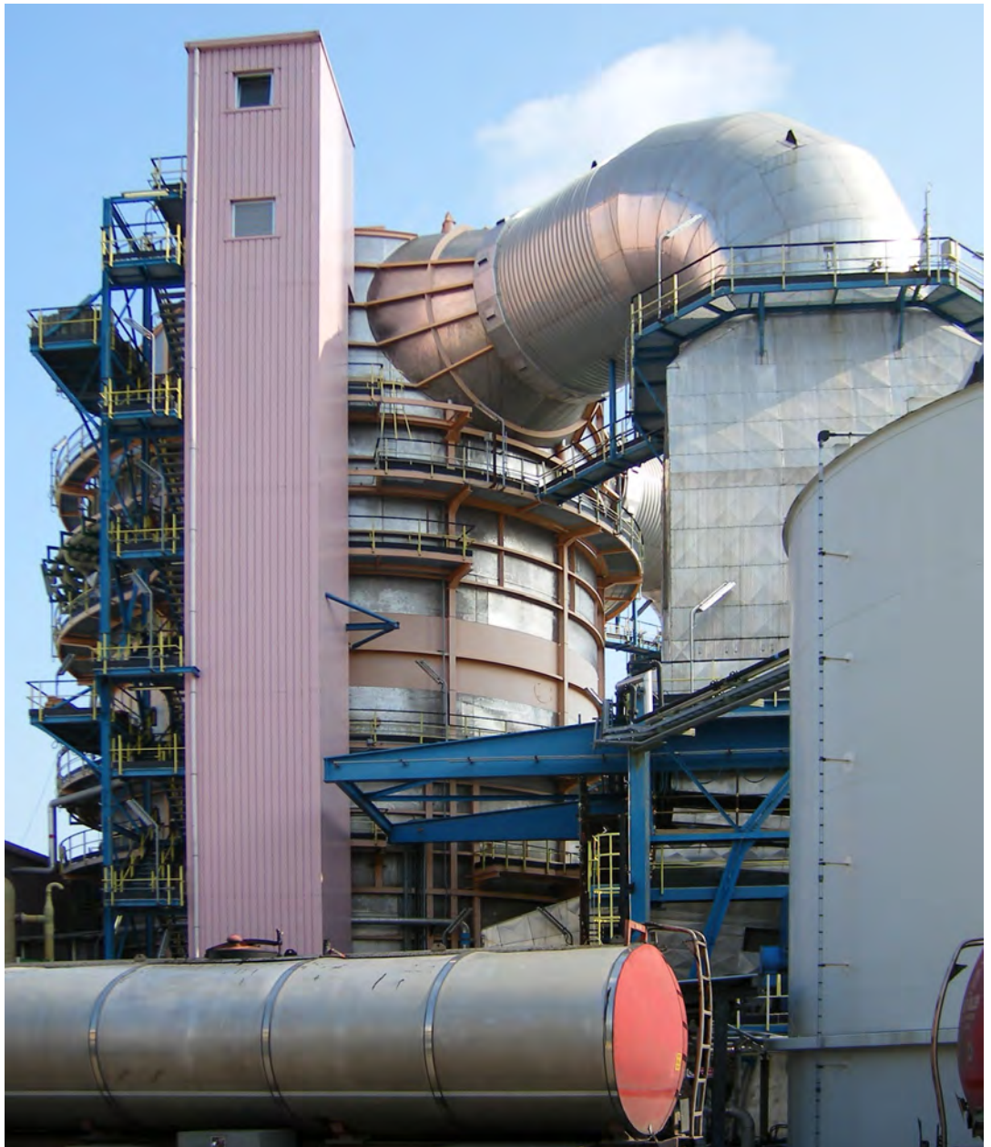
HPASS in a flue gas scrubber application. (Source: Outokumpu)
