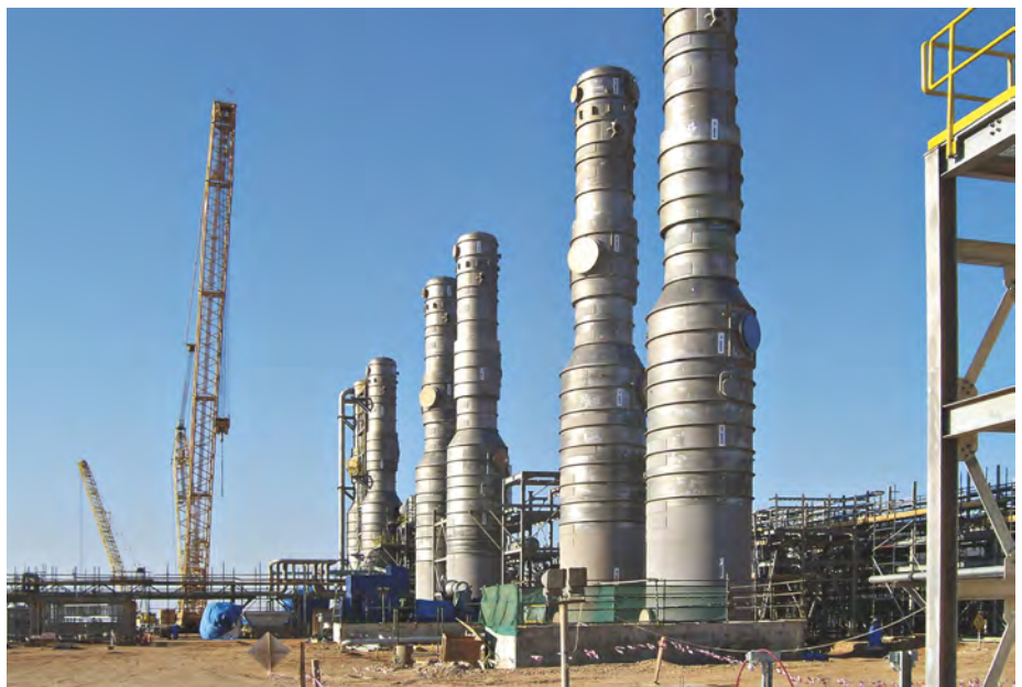
2507 stainless steel enhanced oil recovery equipment. © Aquatech
