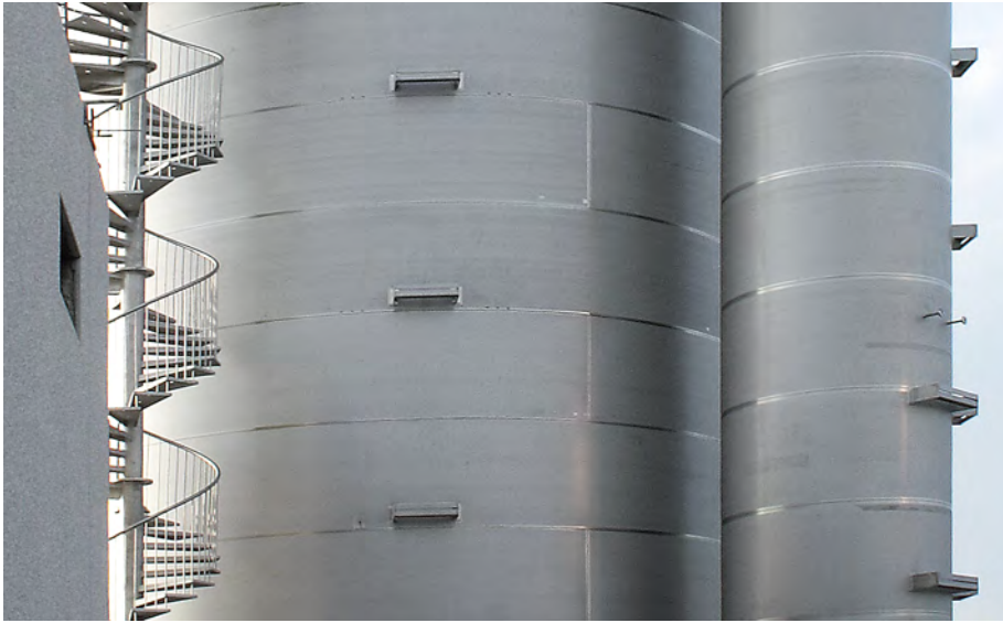
Part of a 31 m (102 ft) tall 2205 duplex stainless steel tank. © Outokumpu
