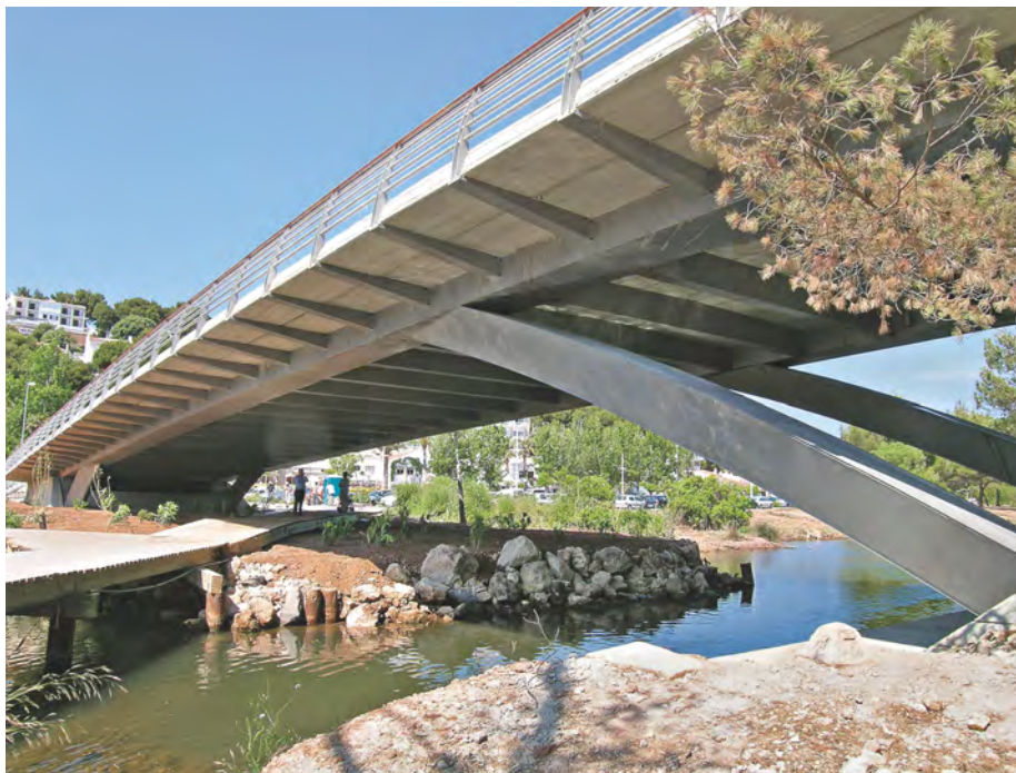
Bridge in Cala Galdana on Menorca fabricated using 2205 duplex stainless steel. © PEDELTA
