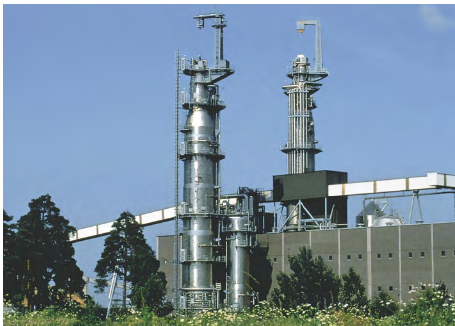
2205 continuous sulphate pulp digester and impregnation tower, Sodra Cell Mönsterås, Sweden. © Kvaerner Pulping
