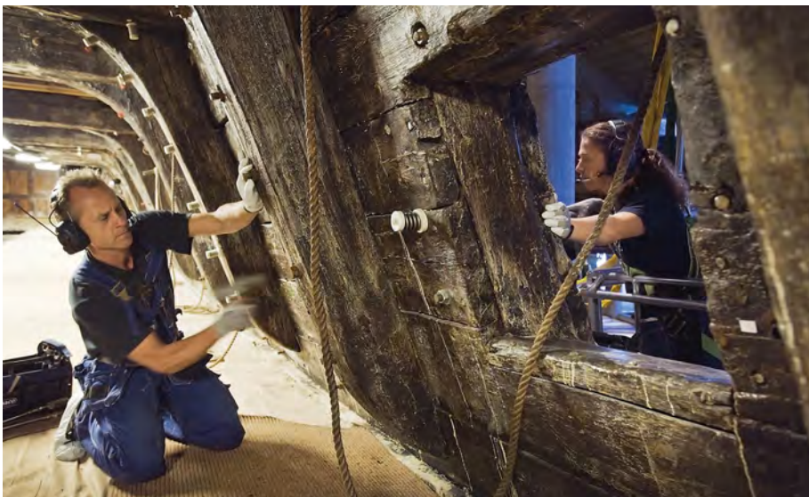
Installation of hyper duplex stainless steel bolts to preserve the historic wooden Vasa ship in Sweden. © Anneli Karlsson, the Swedish National Maritime Museums
