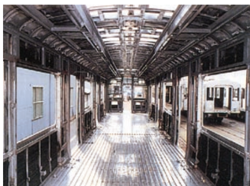
Photo: ArcelorMittal Stainless Belgium, Genk ( B )
