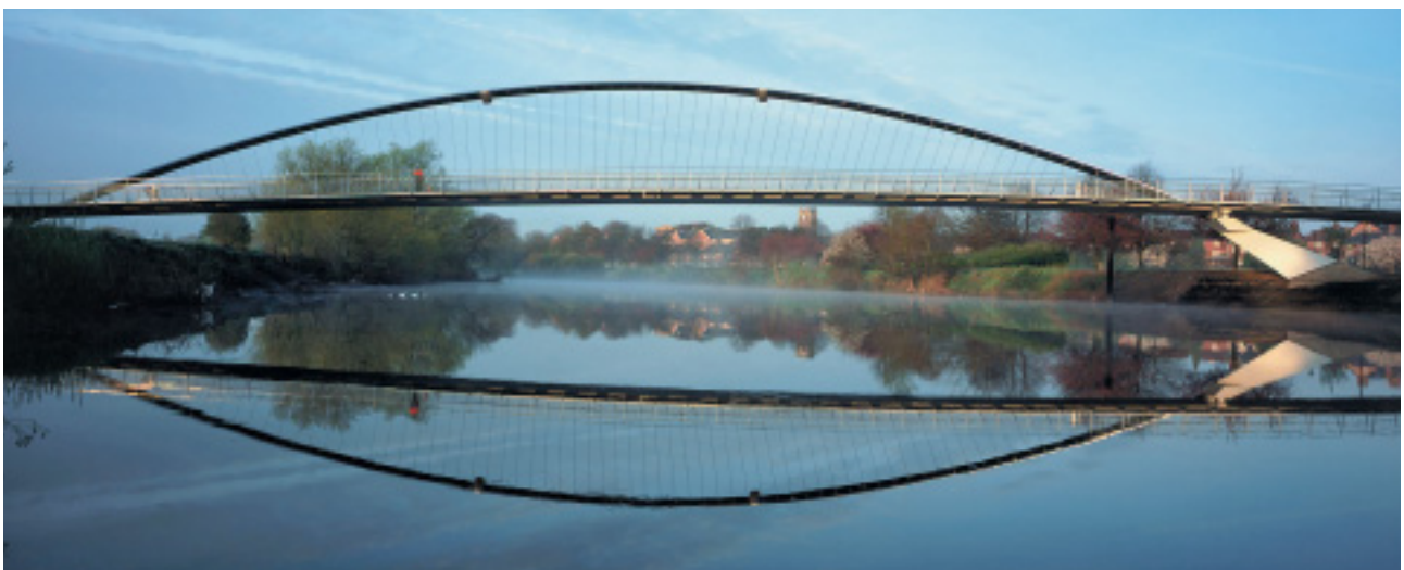
The stainless steel arch, spanning 80 m across the river, is tilted at 50^\circ to the vertical.
