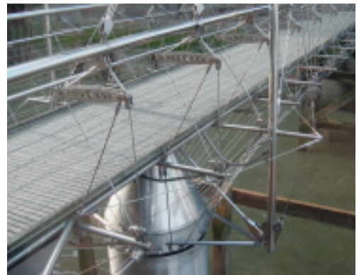
A fan-shaped arrangement of tie rods supports the rotating footbridge.
