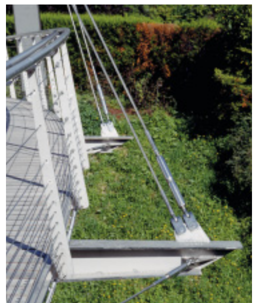
Pairs of tie rods connect the cross beams to the arch.
