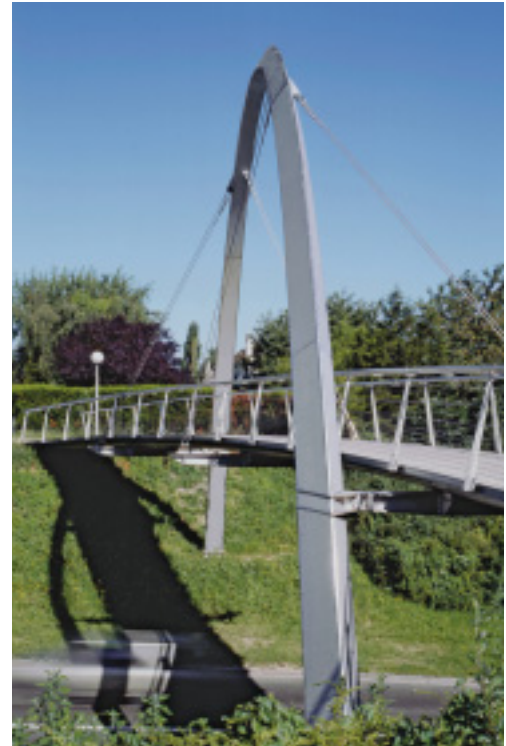
The triangular cross section of the arch tapers from the foundations up to the apex.
