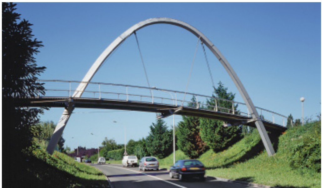
The bridge deck curves underneath the stainless steel arch over a busy road.
