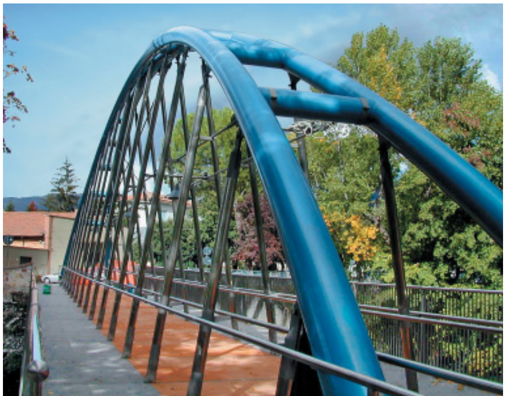
Stainless steel is used for the bridge components subject most to public use and statical loading.
