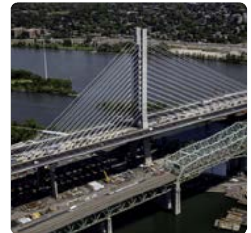
Champlain Bridge, Montreal, Kanada Foto: Infrastructure Canada
