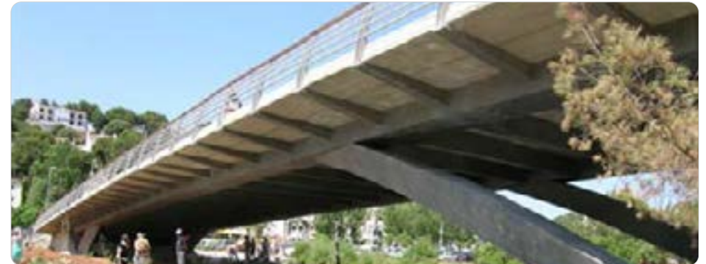
Brücke in Cala Galdana, Menorca
